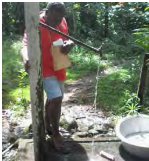
Guadalcanal Provincial Government (GPG) water technician in Vatupilei. Source: Joe Hagabore
